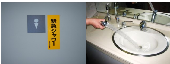
Emergency showers are located in restrooms marked with this sign
